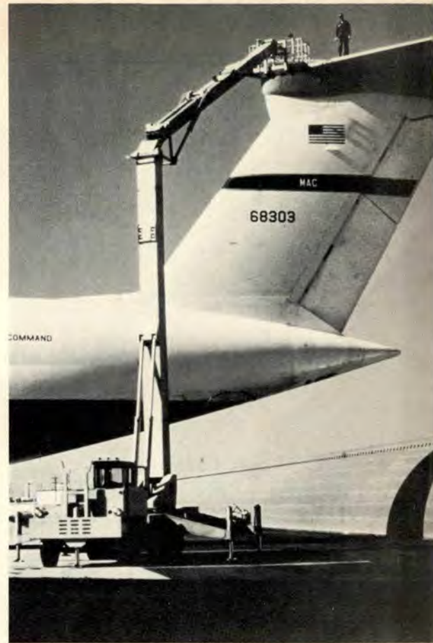
High-lift Calavar is part of AGE for C-5. Horizontal stabilizer is 65 feet above the ground.
